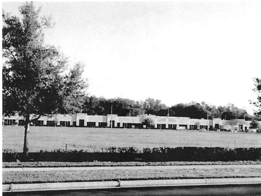
Subject Site, looking north (office uses at northern property boundary)
